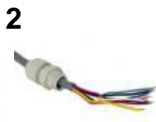
2.- The cable has to be stripped of its jacket for 2 inches (50mm) and the wires need 1/8" (3mm) stripped ends.
